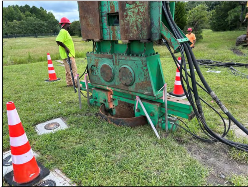
Caisson Installation
