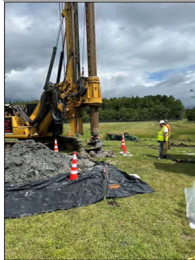
Soil Removal from Caisson Using Drill Rig
