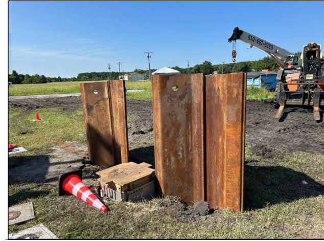
Sheet Pile Installation
