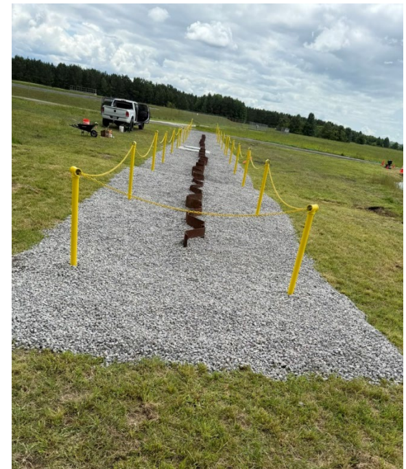
Completed Wall at Surface
