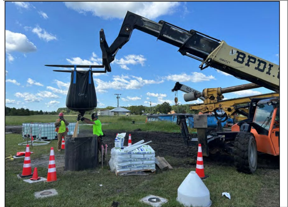
Sand Filter Installation
